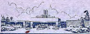
Duarte Road at Myrtle Ave, Monrovia
